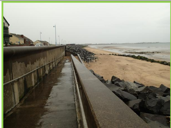
High beach levels almost covering rock bund at access ramp near Little Scar (Asset ref. No. 1221C901C0401C33)
