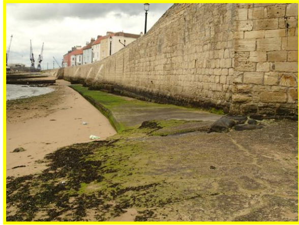
View of Town Wall from east end, showing new toe protection apron (Asset ref. No. 1221C901C0401C35)
