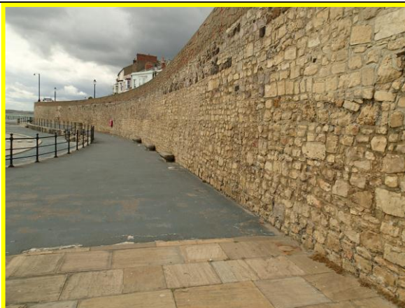
Rear retaining wall at Block Sands. (Asset ref. No. 1221C901C0401C04)
