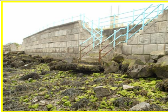
Undercutting of steps and wall near sailing club (Asset ref. No. 1221C901C0401C27)
