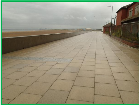
General view of new promenade (Asset ref. No. 1221C901C0501C02)
