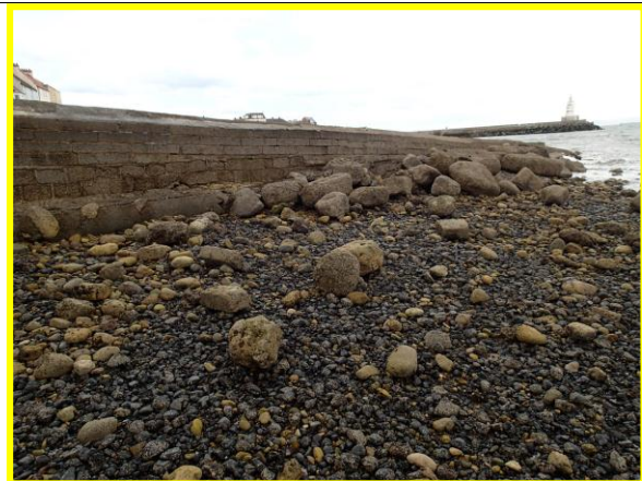
Large groyne structure near mid point of Town Wall marks large change in beach levels, cobble slag beach on west side in foreground. (Asset ref. No. 1221C901C0401C35)
