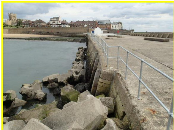
Landwards side of pier showing new handrails. (Asset ref. No. 1221C901C0401C06)
