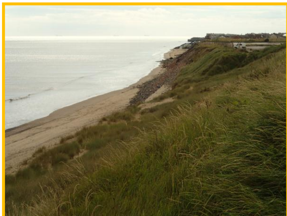
Eroding embankment east of cemetery in mid-distance. (Asset ref. No. 1221C901C0302C01)
