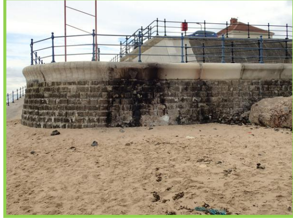
Seawall at return end (Asset ref. No. 1221C901C0303C01)
