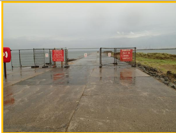
Fencing and warning signs on North Gare breakwater. (Asset ref. No. 1221C901C0502C01)
