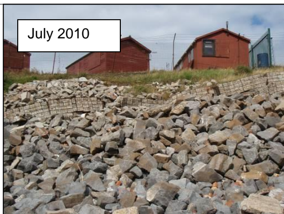
View of Gabion baskets with rock armour. Photo from 2010 report. (Asset ref. No. 1221C901C0401C17)
