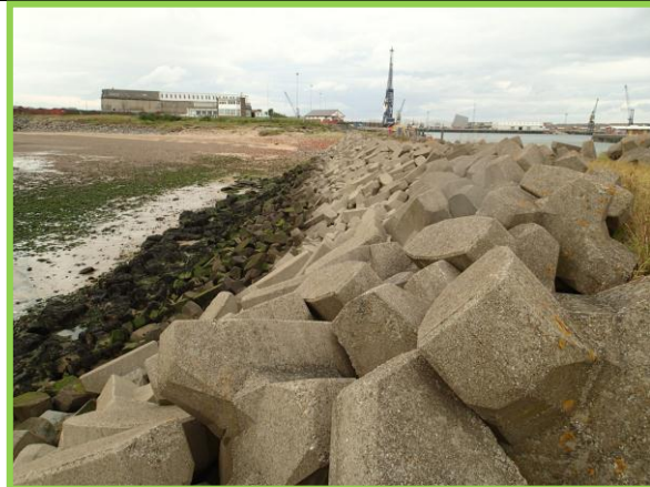
Middleton Jetty in good condition. Retains sand and rubble beach to south (Asset ref. No. 1221C901C0401C16)
