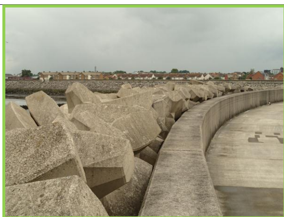
South Pier Accropode armour on outer face (Asset ref. No. 1221C901C0401C32)
