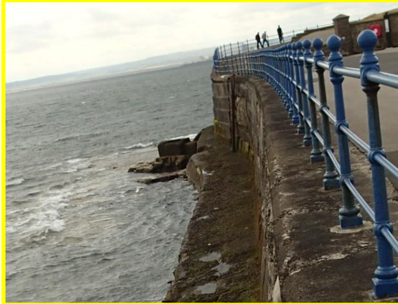
Stepped wall at apex of Headland.(Asset ref. No. 1221C901C0303C03)
