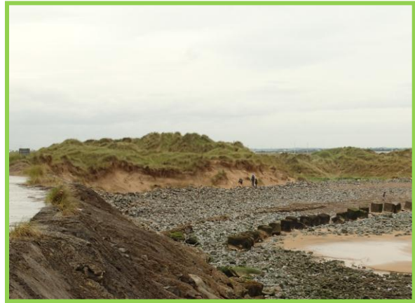
Localised cliffing of the dunes immediately north of North Gare, adjacent to rubble revetment placed to manage outflanking. (Asset ref. No. 1221C901C0502C01)
