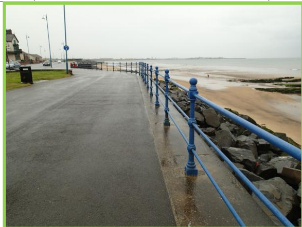
General view of promenade in good condition (Asset Ref. No. 1221C901C0501C05)
