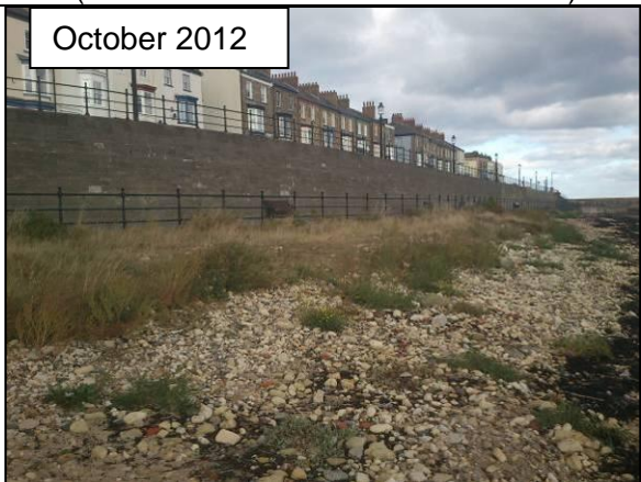
High cobble beach at mid-length of wall (Asset ref. No. 1221C901C0401C05)
