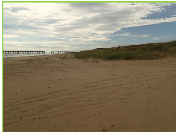
Wide beach at North Sands adjacent to former Britmag site. (Asset ref. No. 1221C901C0302C01)
