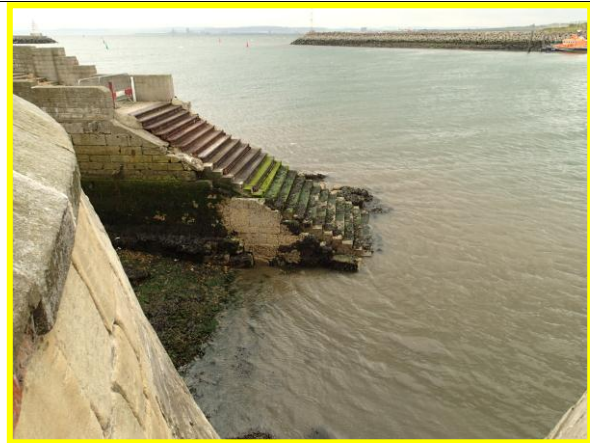
Steps at former passenger ferry landing at west end of town Wall, (Asset ref. No. 1221C901C0401C35)
